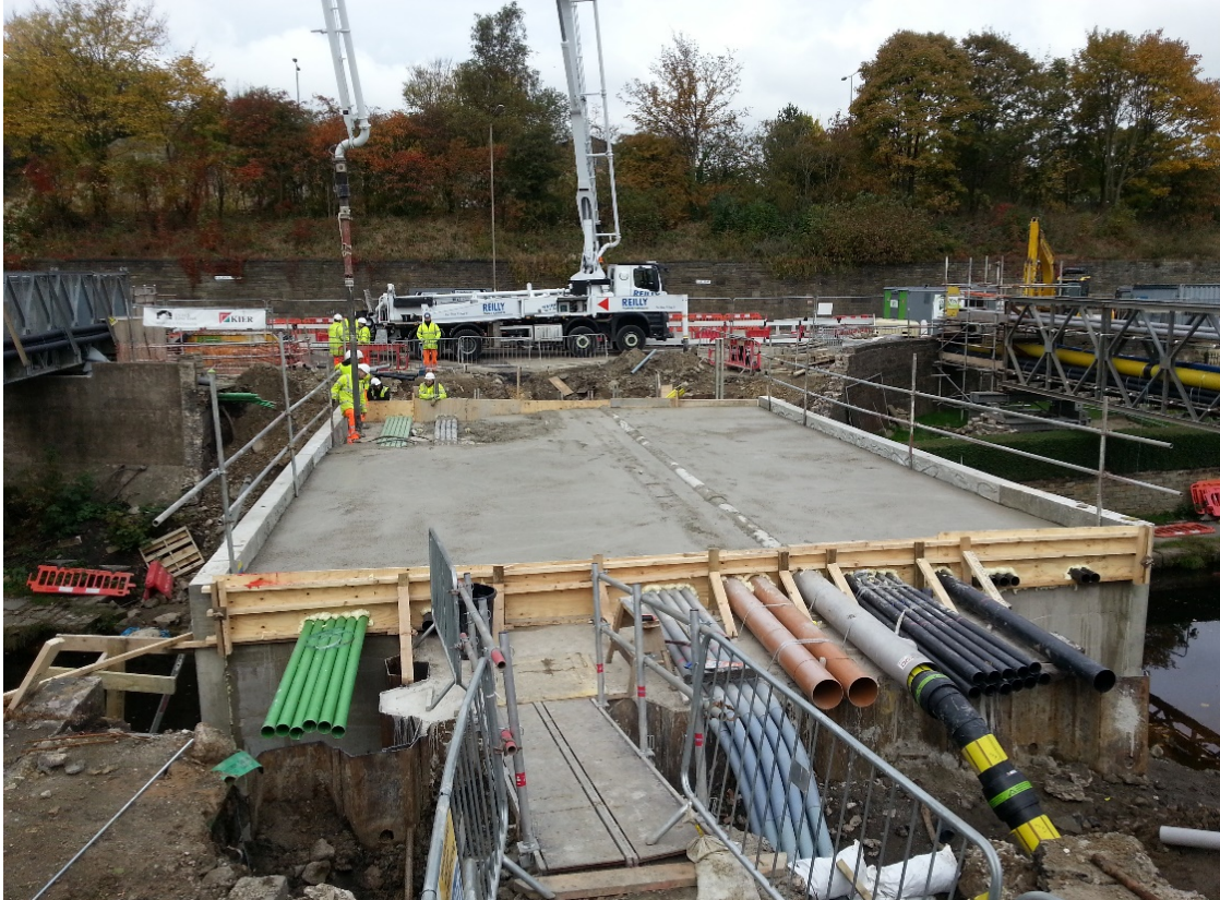
Plate 2: Elland Bridge Calderdale during its reconstruction following Storm Eva. Note the multiple aligned service conduits being built into the ‘bottleneck’ structure. (Image courtesy John Lamb, 2017)
