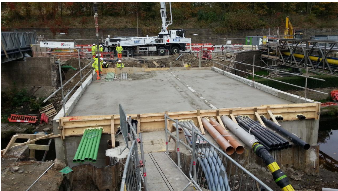
Image: Elland Bridge, Calderdale — reconstruction following Storm Eva, Boxing Day 2015. © John Lamb
