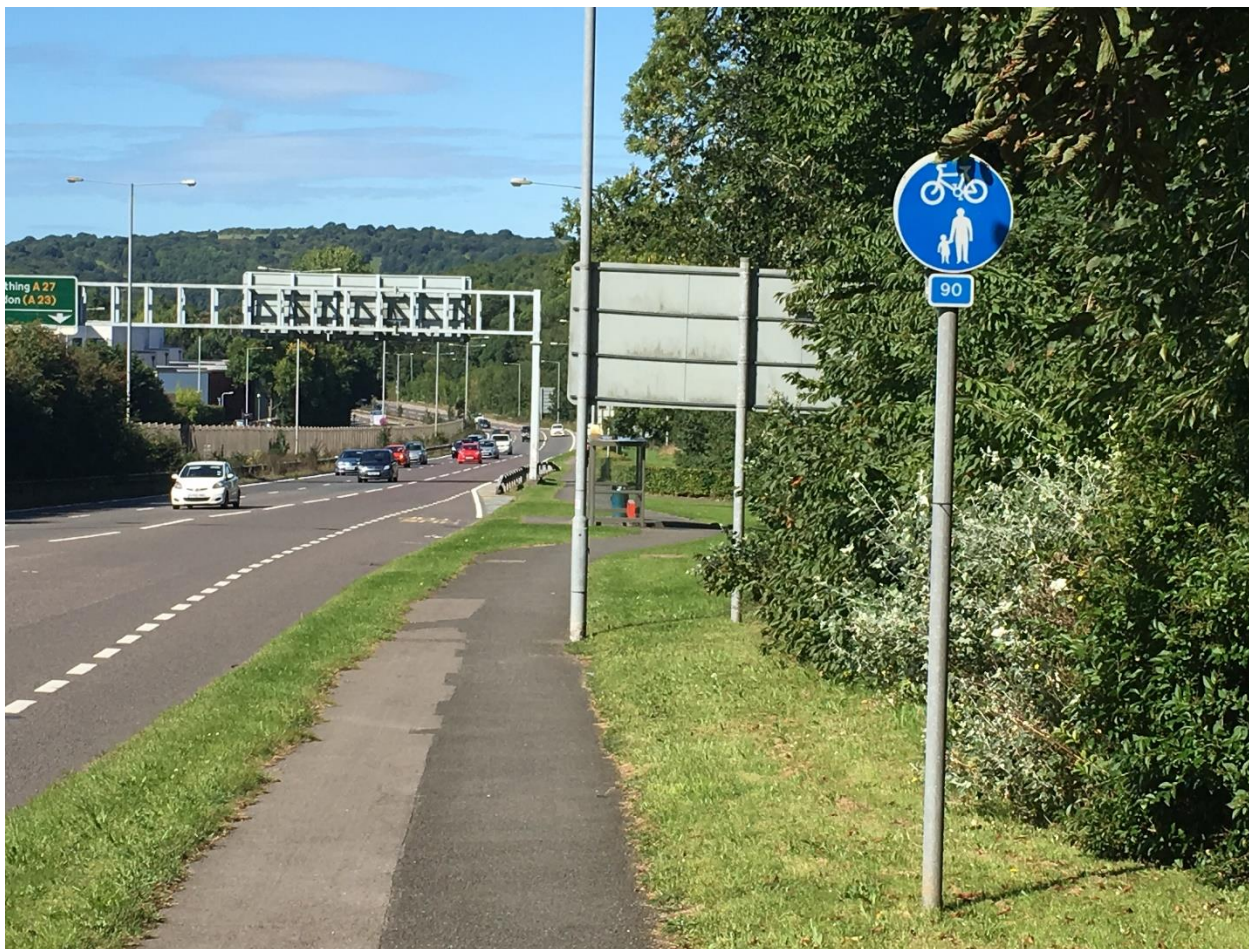
Photo 7: Unsegregated Shared Use Cycletrack/Shared Footway and Cycletrack
