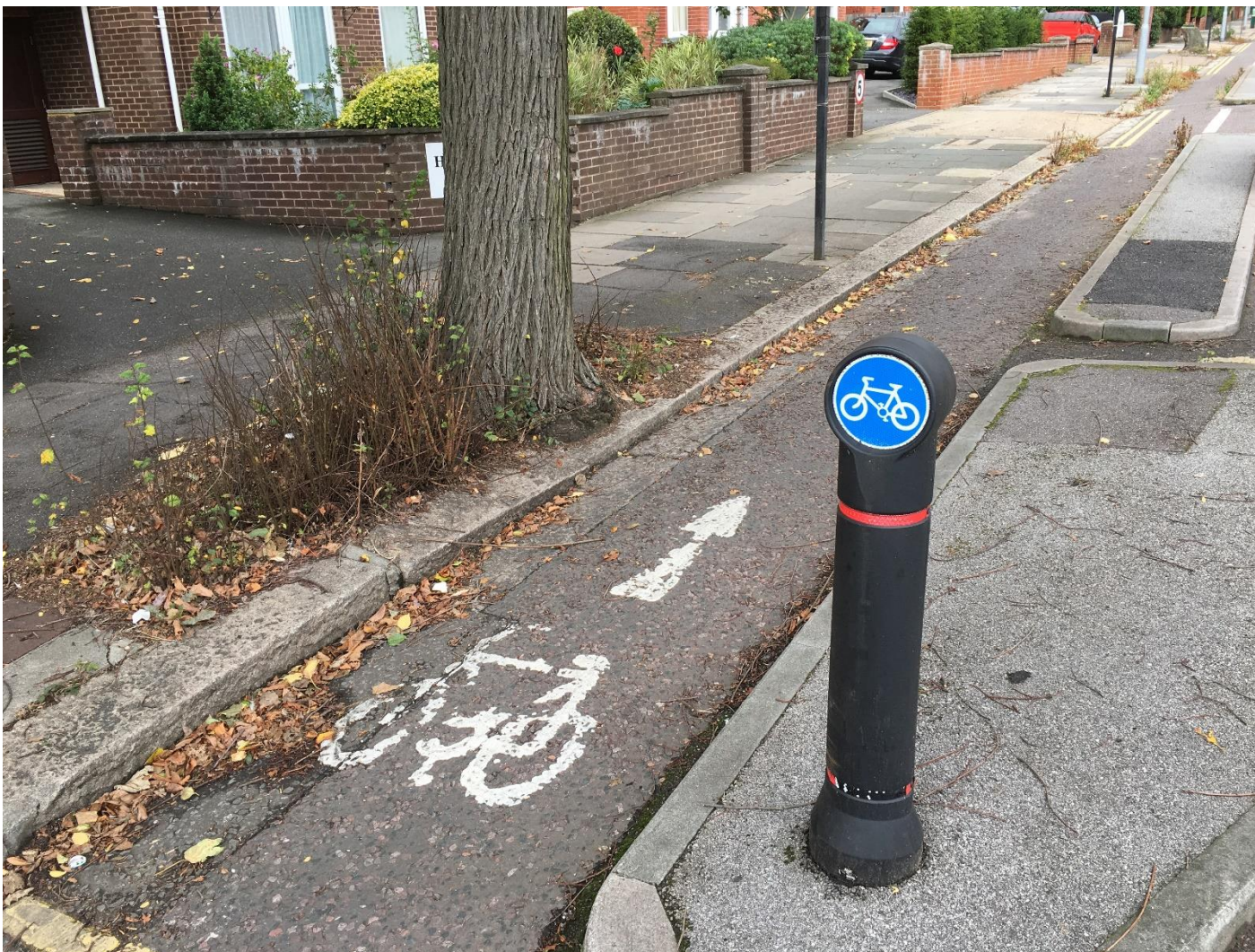
Photo 4: Cycle Track at Carriageway Level with Physical Separation
