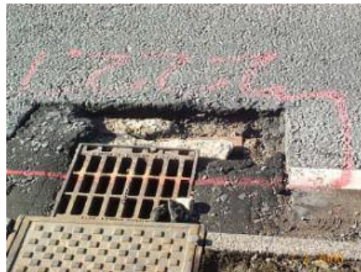
Damage to ironworks, image courtesy of Atkins
