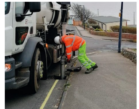
↑ Gully emptying in progress
