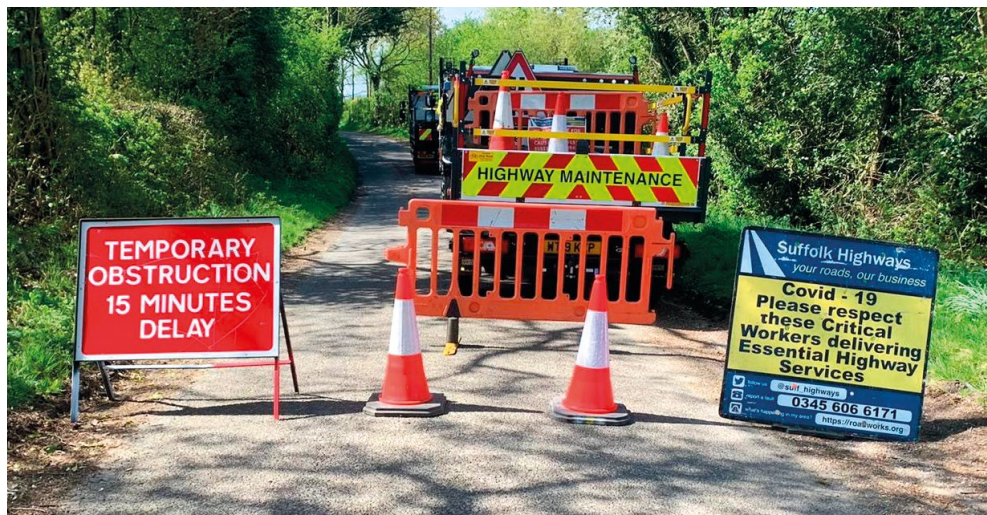
↑ Extra signage has been used by Suffolk Highways in recent weeks to keep the public informed
